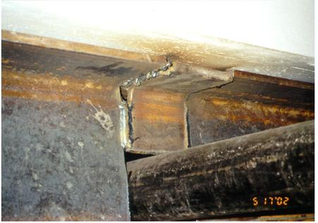
A photograph showing a large pipe passing through a steel beam connection. The pipe is positioned such that it interferes with the structural integrity of the joint. A date stamp '5 17 02' is visible in the bottom right corner of the photo.
