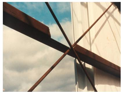
A photograph showing a steel beam with a diagonal brace. The brace is positioned such that it interferes with another steel beam, creating a complex structural situation.
