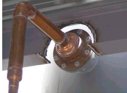
A photograph showing a pipe that has been bent at an angle to clear a steel beam. The pipe is supported by a circular metal plate with bolts, which is attached to the steel structure.
