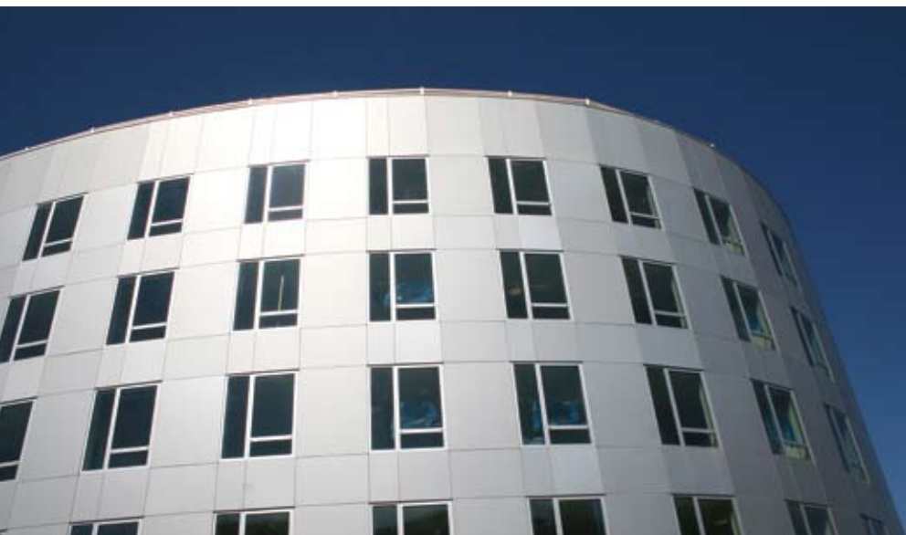
Curved metal panels (above) alternate with red brick to provide visual transition points between the interconnected buildings.
