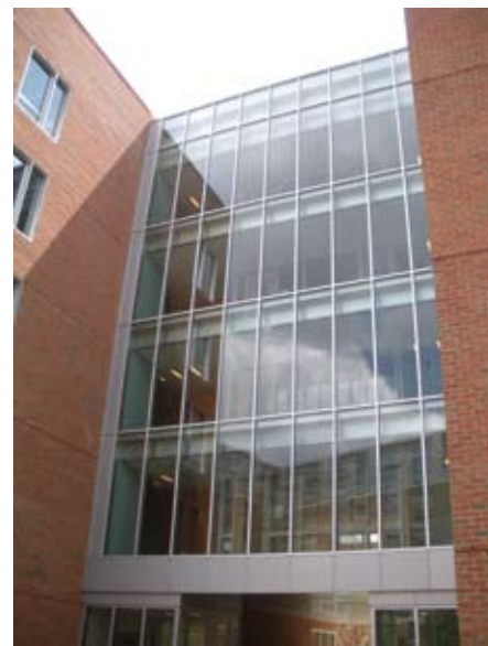
A pedestrian bridge with a curtain wall links two buildings within the complex.
