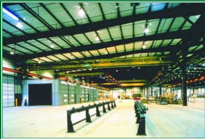
Shown at top is the Transcrypt building in Lincoln, NE, while pictured above is the interior of the Wilkof-Morris plant in Canton, OH.
