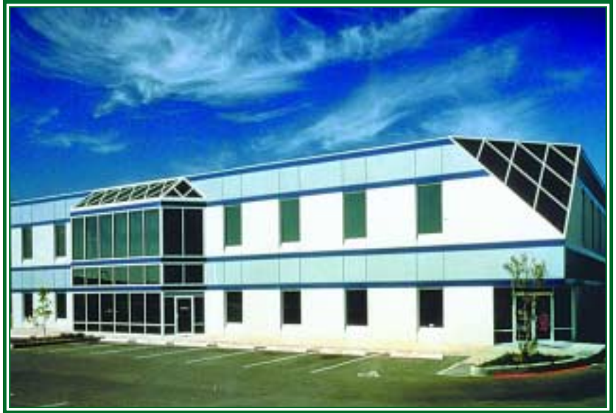
Leon's Carpet & Tile headquarters (above) in Austin, TX, and the Gold Shore Casino (opposite) in Biloxi, MS, demonstrate the versatility of today's metal buildings.
