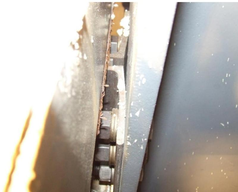
Figure 8.17: Photograph showing prying action occurring at connection
