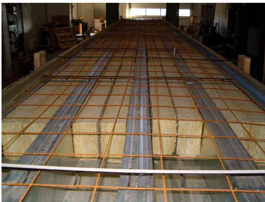
Figure 7.6: End view of RW-DD System prior to concrete pour showing mineral wool placement
