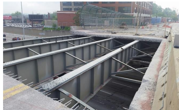
Figure 7: Phase 1 of the Span 2 Repairs with Deck Removed.
