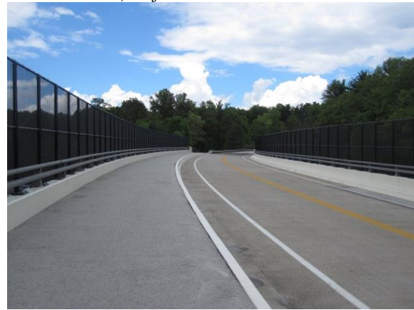
b) After Rehabilitation
