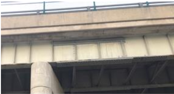
Figure 6: Span 1 Repairs Installed in Fascia Girder.
