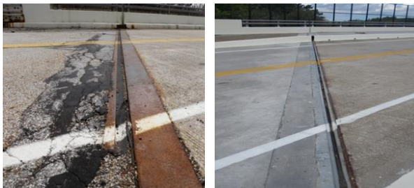
Figure 18: Expansion Joint Replacement (existing at left, new at right).
