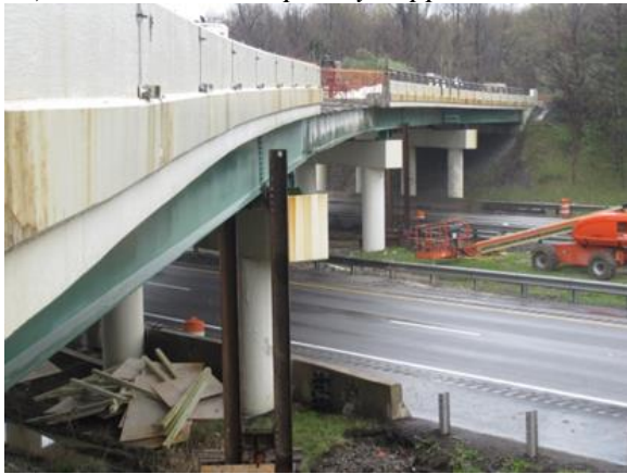
b) Field Photo Showing Temporary Support Locations
