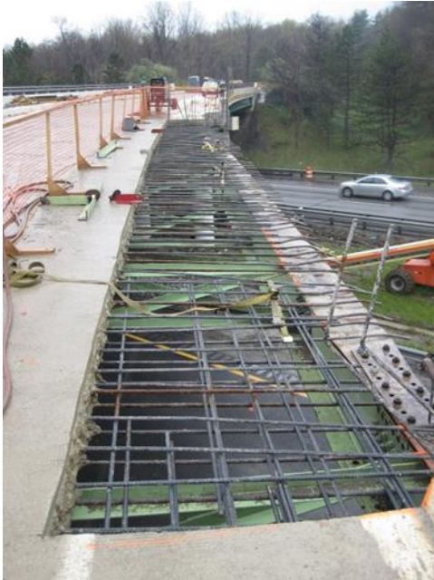
Figure 15: Deck Removed, Existing Beam Still in Place.
