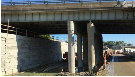
Figure 3: New Pier 1 Constructed to the West (left) of the Existing Pier 1.
