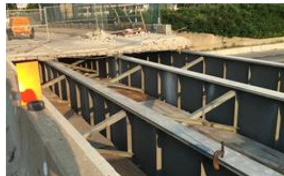
Figure 8: Phase 2 of the Span 2 Repairs with Deck Removed.
